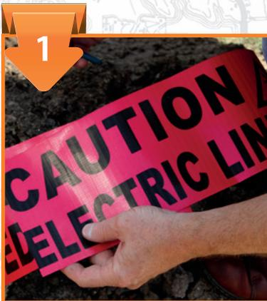
Overlap two ends of detectable tape being spliced by 6-10 inches.
