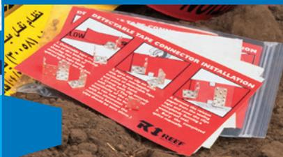
*Terra Clips can be used to connect the ends of each roll, tee or lateral for easier location and for connecting conductively to the foil in the tape.*
