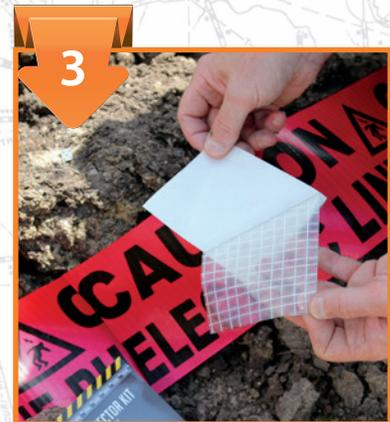
Remove the release paper from the adhesive sealing tape.
